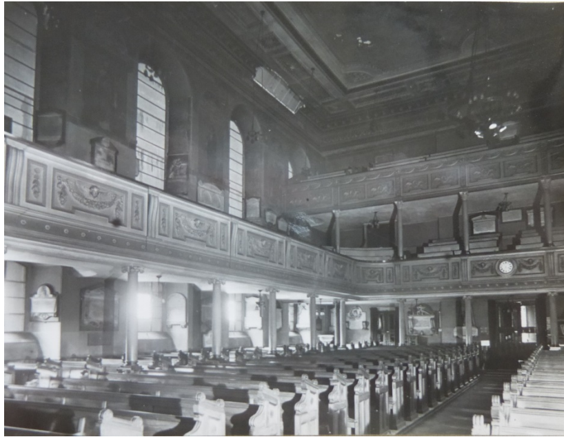
1943 photograph showing war damage to windows and fabric and the frescoes painted by Edward Armitage, RA at first floor gallery level
